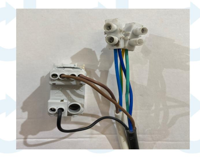
The BLACK and BROWN wires coming from the motor are directional wires, so may need to be swapped over if the operational direction is incorrect. (i.e up button taking the door down & vice versa)
